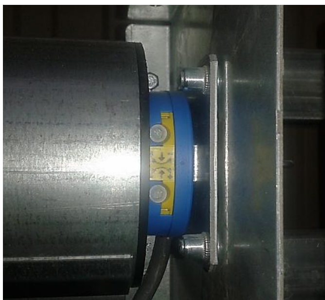
Pic. 1 Limit switches of the curtain engine (upper and lower position).
